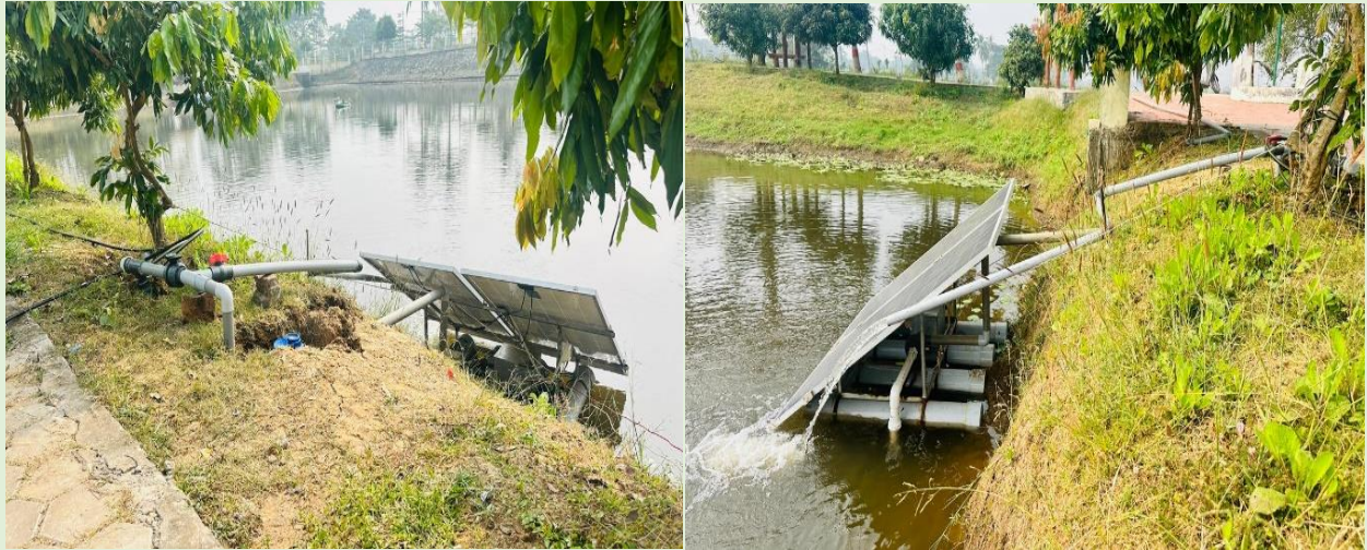
Fig.4. The floated solar pumping unit in operation
