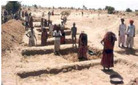
Fig. 3.34 Borrow pit in dryland area before plantation
