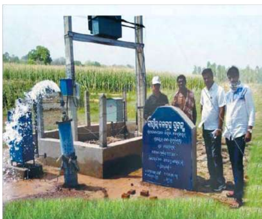
Fig. 3.13 Deep tube well
