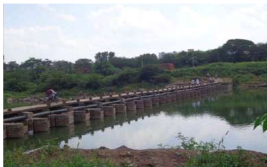
Fig. 3.46 Bandhera on Bheema river
