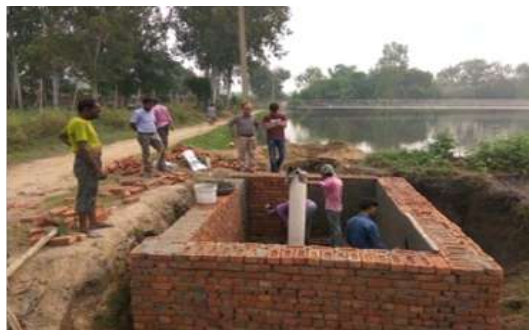
Fig. 3.49 Percolation tank Source: Authors' own collection
