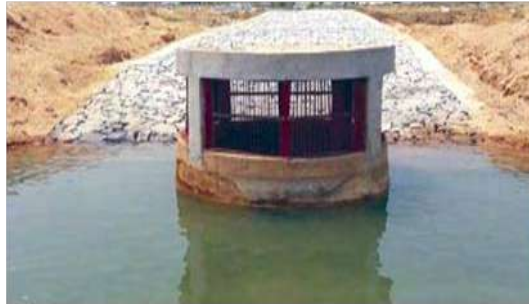
Fig. 3.17 (a) Mega lift irrigation system
