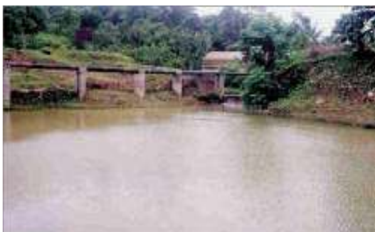
Fig. 3.38 Construction of runoff water collection ponds
