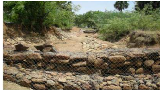
Fig. 3.33 Gabion structures in waterways
