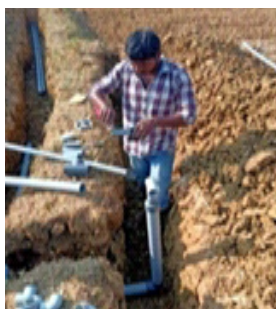
Installation of drip irrigation system at Badakusunpur
